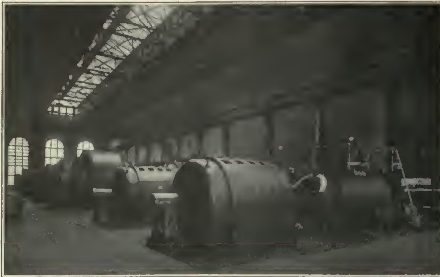
FIG. 488. POWER STATIONS. Interior View, Power Station of the Pennsylvania Railroad, New York City. Capacity 32,500 kw. for Traction and 6,000 kw. for Lighting.
